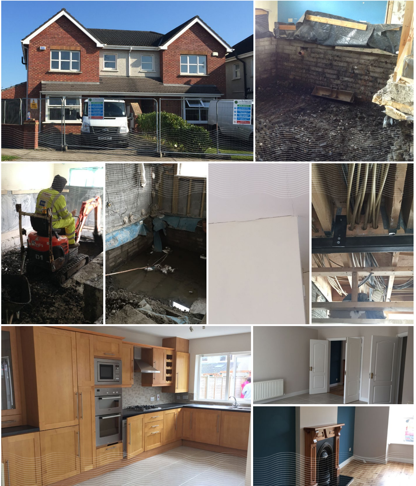
Pyrite remediation work in 2015
