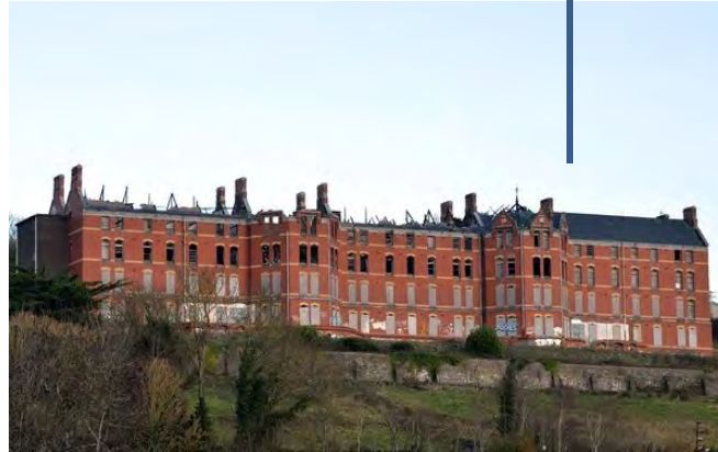
Cork, St Kevin's Former Hospital
