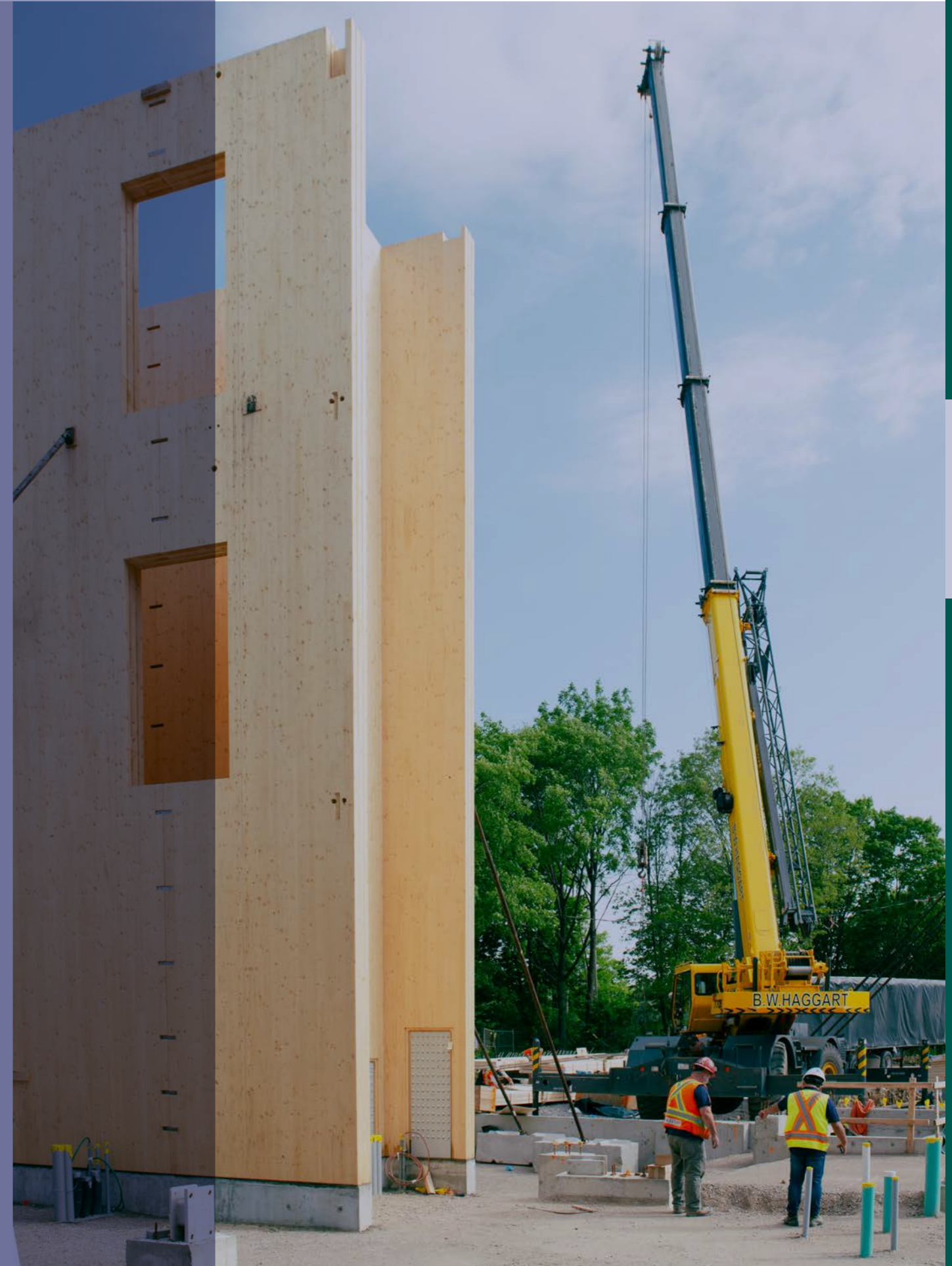
Installation of CLT core - Bucholz McEvoy Architects / Kris Gurner
