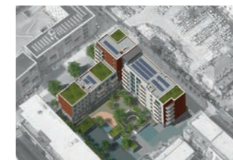
Case Study 15 Railway Court, Dublin
