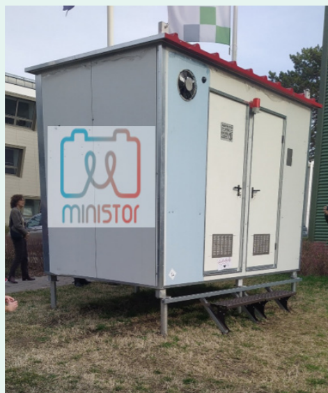
Example of thermal energy storage in a mini sized container, as part of the Horizon 2020 project Minister
