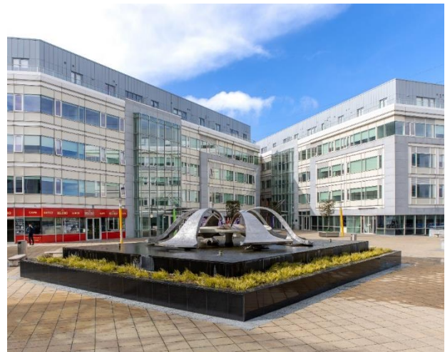
Park West Plaza after the office-to-residential conversion
