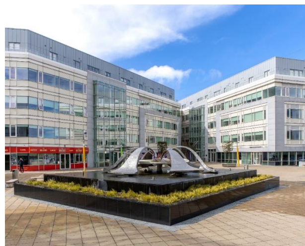
Park West Plaza after the office-to-residential conversion
