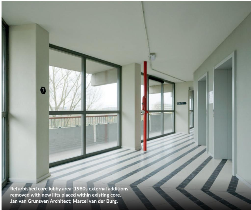
Refurbished core lobby area: 1980s external additions removed with new lifts placed within existing core.
