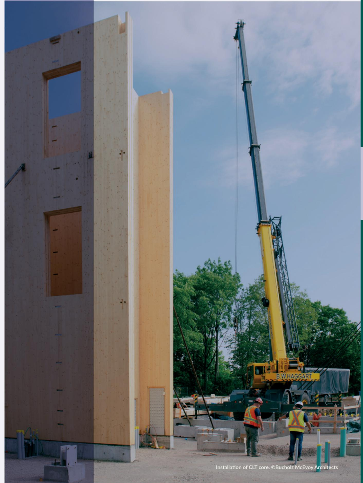
Installation of CLT core. ©Bucholz McEvoy Architects
