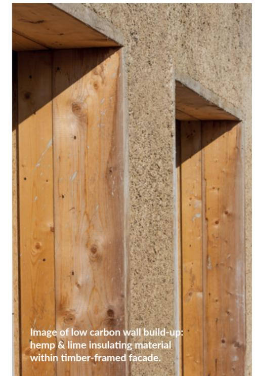
Image of low carbon wall build-up: hemp & lime insulating material within timber-framed facade.
