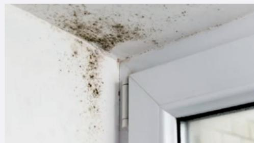
Example of mould growth at window resulting from poor ventilation.
