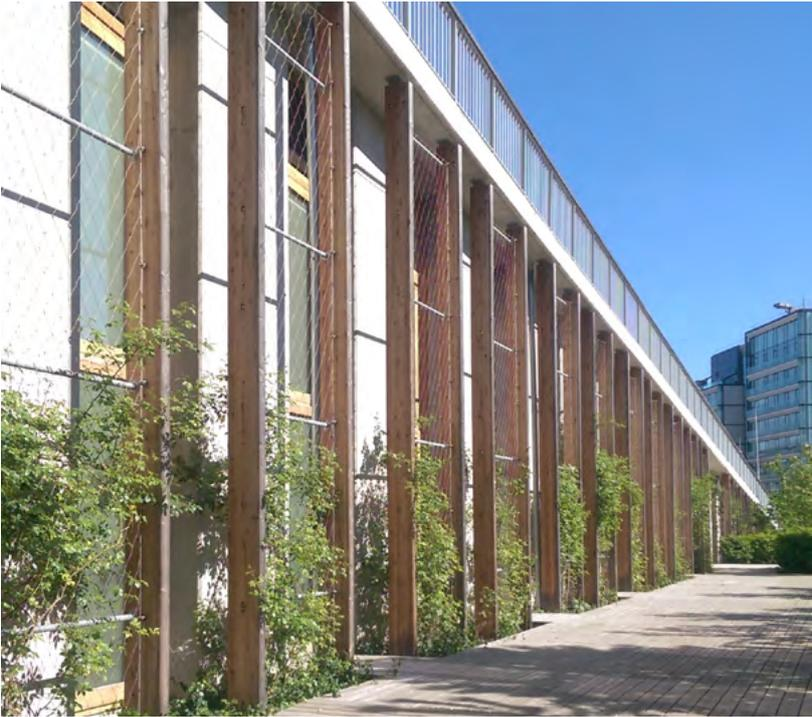
**Image showing green screen in ground floor units.**
