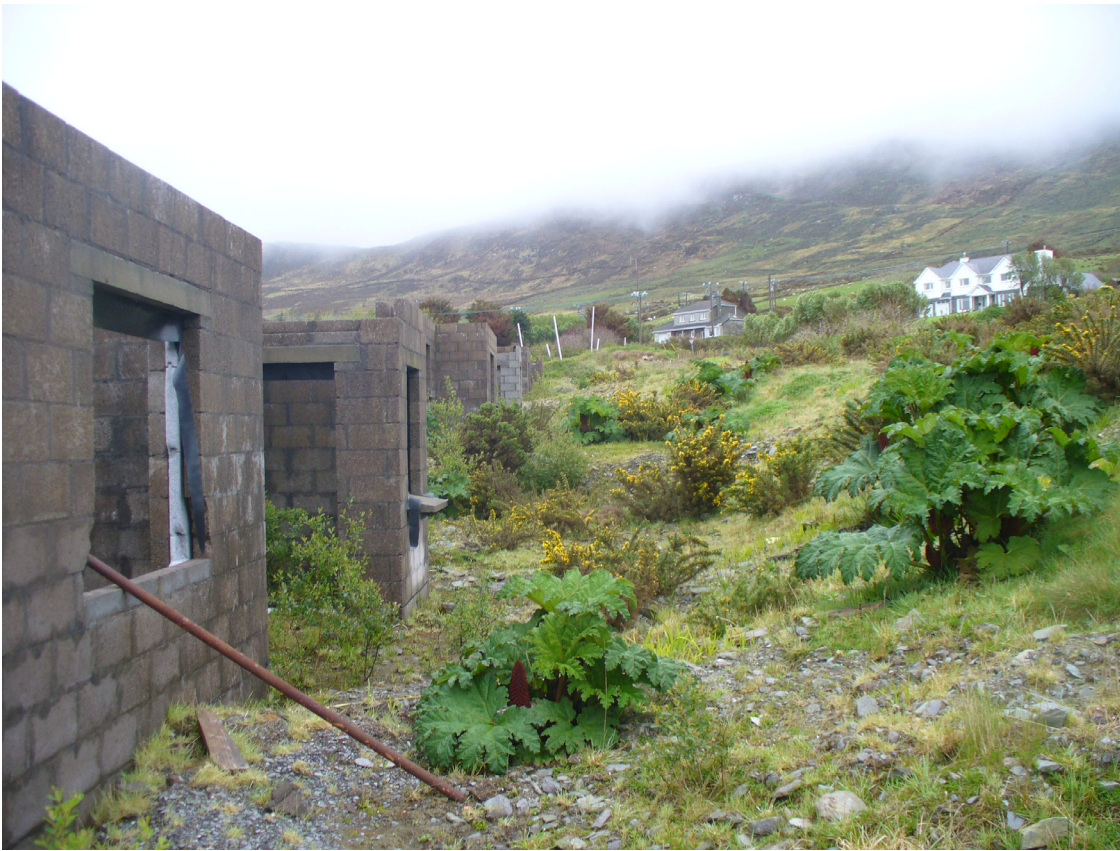
These images illustrate progress under the SRF Lighthouse View, Caherciveen, Kerry, Before/After Resolution
